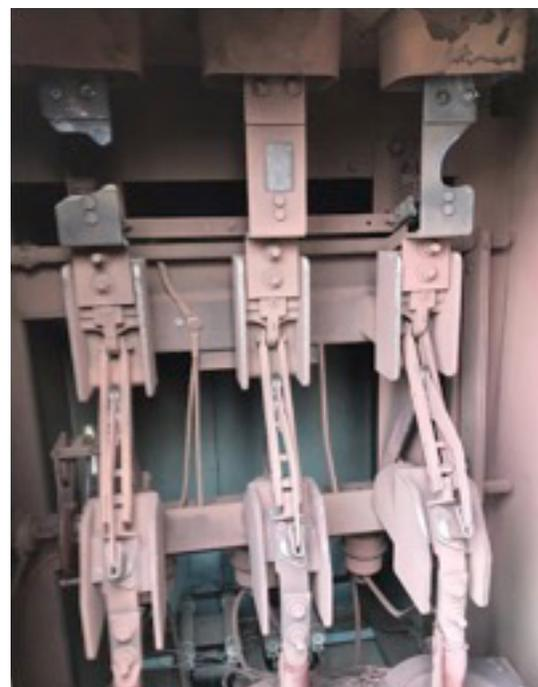
Figure 1 – Image of failed incoming switch
