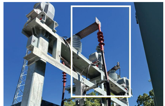
Figure 1: Equipment with elevated levels of total harmonic distortion
